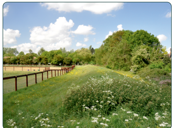
Photo D6. Flood embankment
