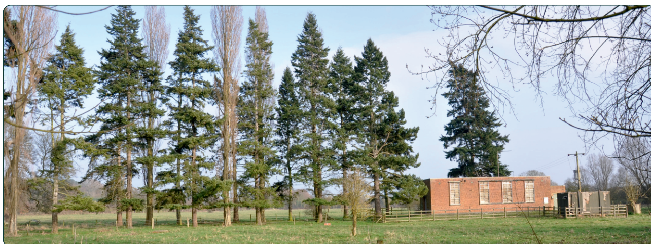
Photo F3. Eastern Pumping Station
