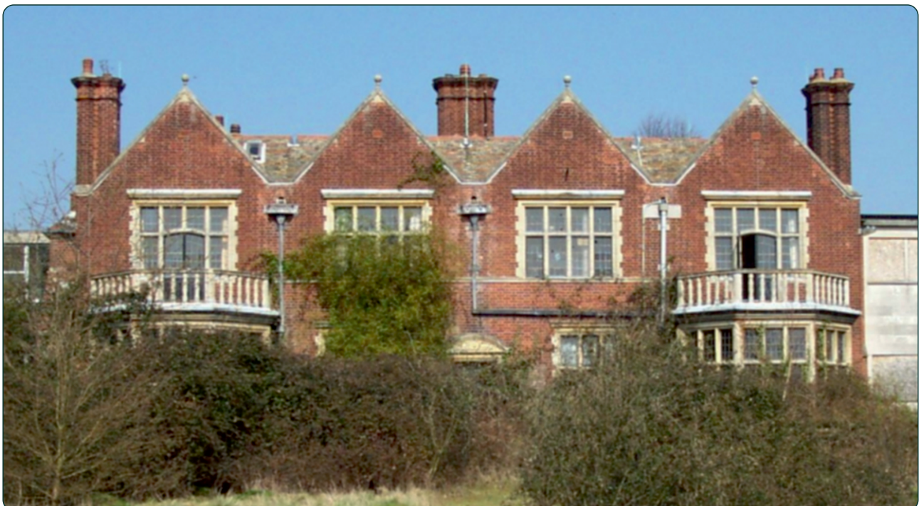
Photo E2. Rear elevation of Houghton Grange
