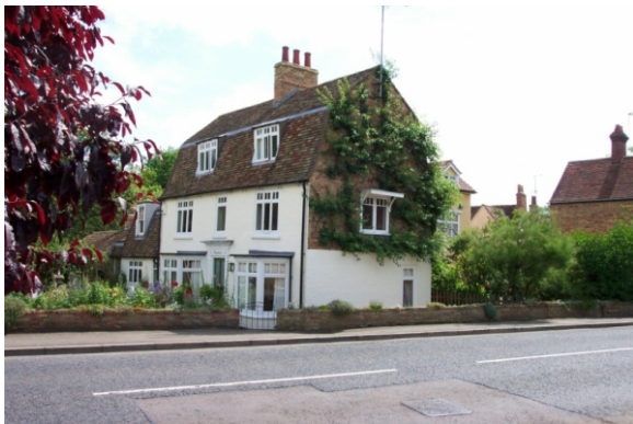
No. 13 Thrapston Road - Grade II Listed Building.
