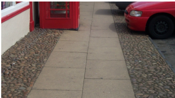
Along High Street there is a distinct character to the footpath: cobbles in the footing of buildings and the road with York paving set down the centre.
