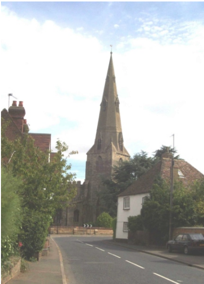
The spire of the church is the key focus looking down Thrapston Road. Vegetation in gardens and the church yard contribute to this view.
