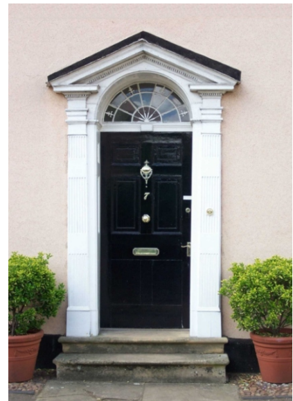
No 7 East Street has a fine classical door with pediment casing and fanlight.
