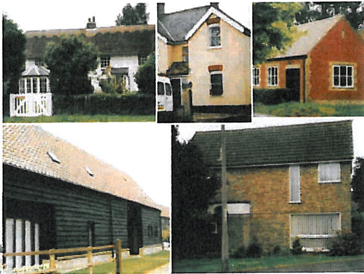
Some building exteriors showing various roofing materials
