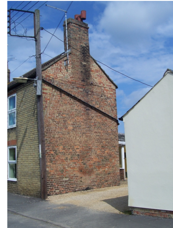
19 Rectory Lane shows possible evidence that it has been refronted and that the original mansard roof has been raised. Although the property is not listed, it is classified as a Building of Local Interest.
