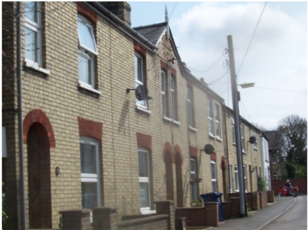
O - 1-15 Rectory Lane
