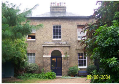
V. County Gaol Watchkeepers House
