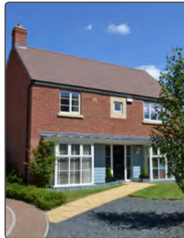
Large ground floor windows enliven this house
