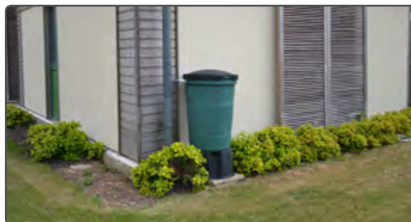
Water butt - rainwater harvesting
