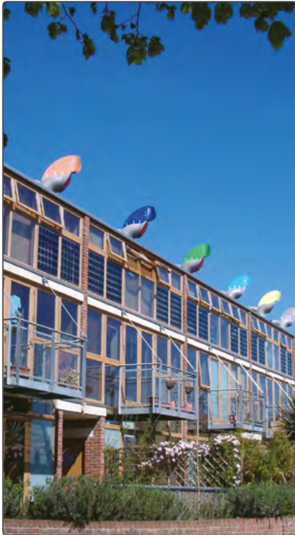
The amount of glazing on this building maximise the natural light into it
