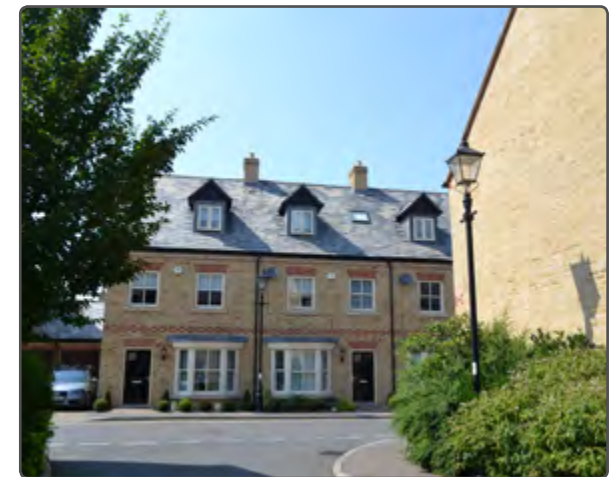
This elevation is animated with bay windows - Huntingdon
