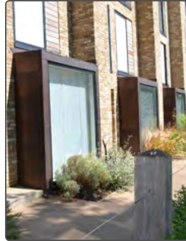
This corten steel window has a deep projection that adds interest to the building
