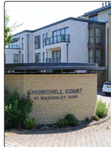
Well ventilated bin store
