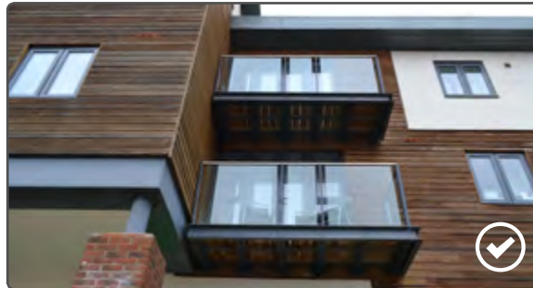
Deep external balconies
