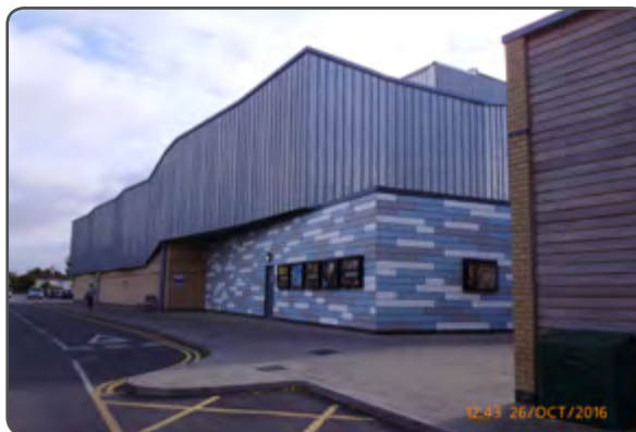
Scale and mass of the cinema building broken up through use of subtle variation in height, undulation on external cladding and different use of materials and colours, Rowley Arts Centre, St Neots
