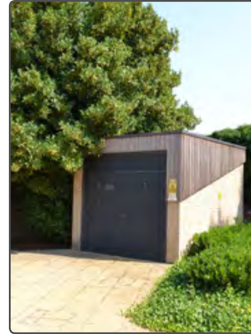
Substation clad in contemporary design
