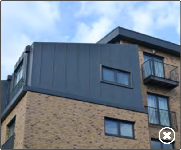
This material is a poor substitute for real metal standing seam
