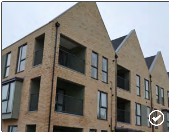
Substantial internal balconies
