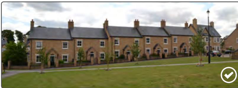
Stepped terrace responding to slope and creating level thresholds to each dwelling
