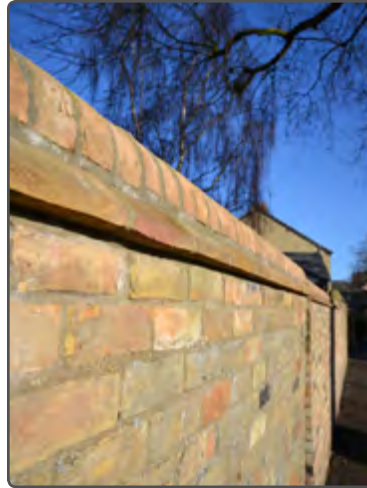
Well detailed brick wall
