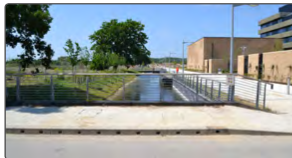
The stream is canalised at this point
