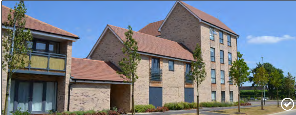
This is good example - the single storey bin store has been incorporated into the building
