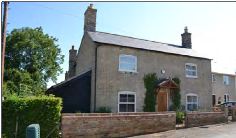
This simple lean to extension fits in very well - Fenstanton
