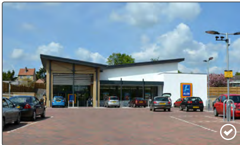
Well proportioned and lively front elevation to this shop - Ely
