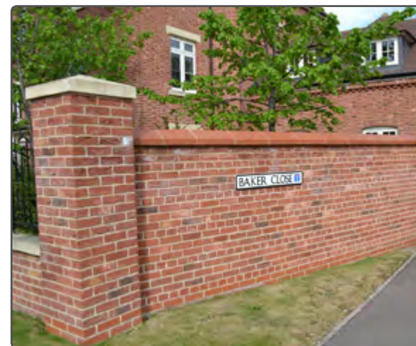
This wall is well detailed and finished - Brompton
