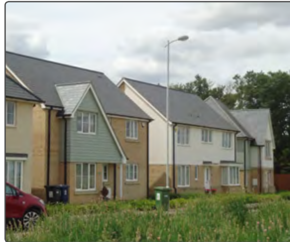
Slate roofing on a contemporary development at Loves Farm, St Neots
