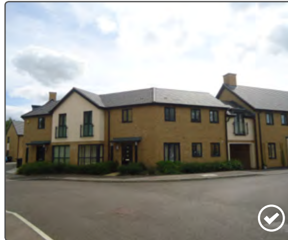
Successful building frontage - Little Paxton
