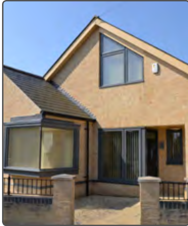
The interplay between windows set in a reveal and boxed windows is appealing here
