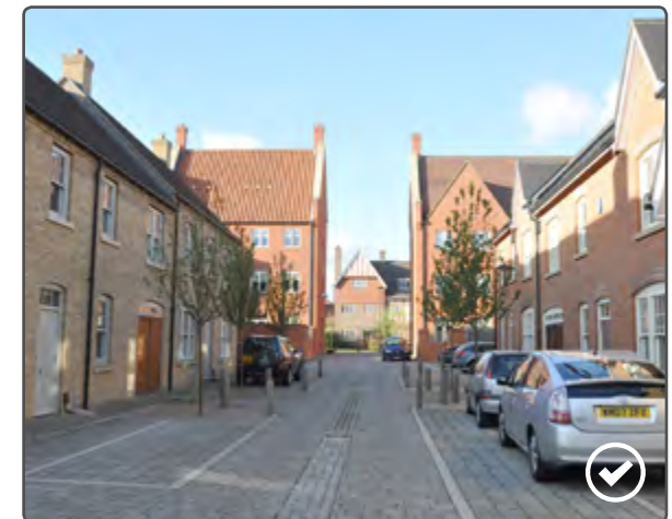
In this high density area car parking spaces are identified by the use of different materials
