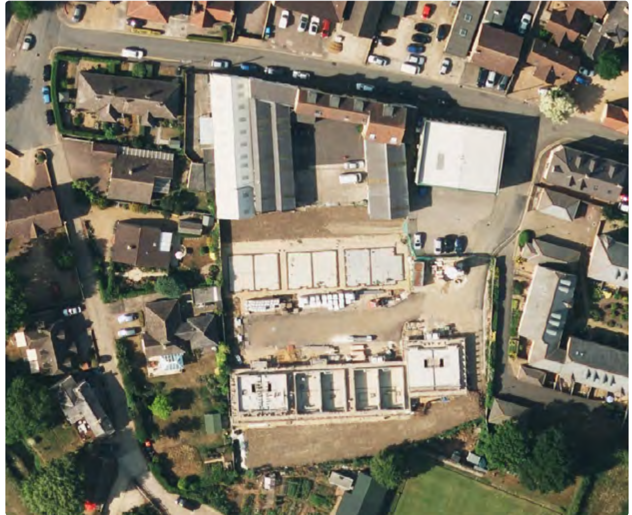
Small group under construction in St Ives
