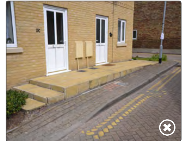
This example shows a building threshold that has not been thought about until the end
