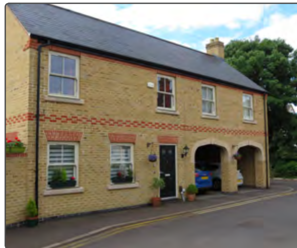
Slate roof at Temple Close, Huntingdon
