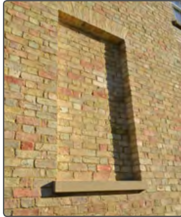
A simple bricked in dummy window with a reveal can add relief to a wall - Huntingdon
