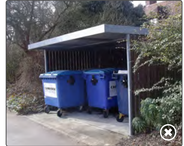
This bin store does not hide the bins very well
