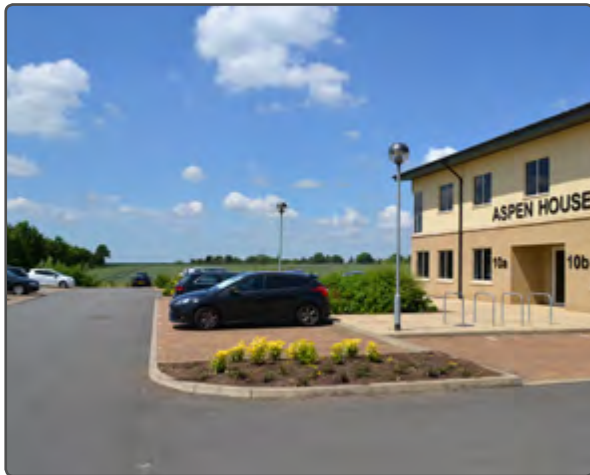
Setting the car parking away from the office building helps to create a pleasant working environment - Huntingdon
