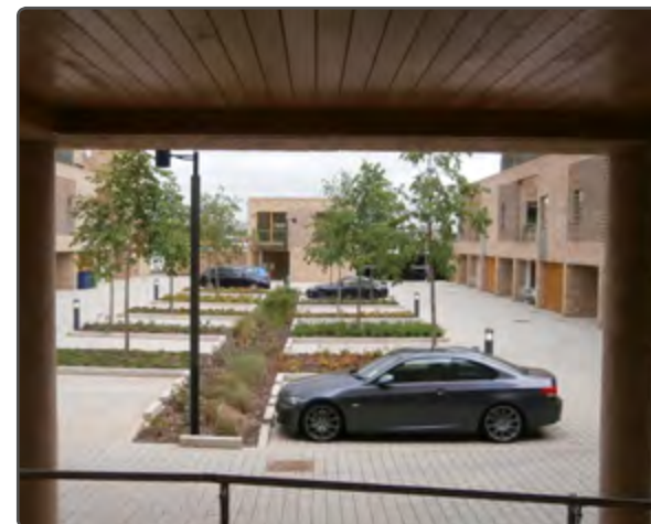
This recent development has provided for generous planting areas between parking bays
