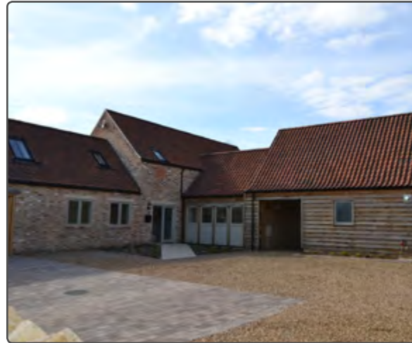
New courtyard development in Great Gidding
