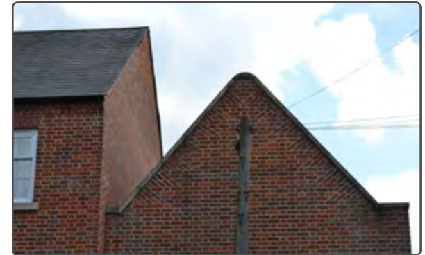
Tumbled brickwork
