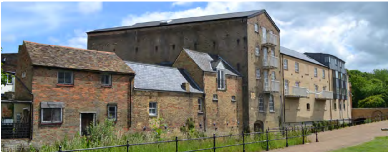
Reuse of former mill building and reinstatement of 3 and 4 storey development adjacent to Hen Brook
