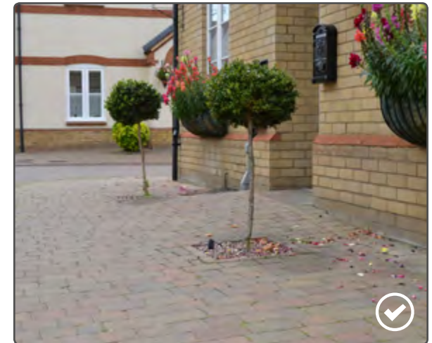
The building threshold is well detailed and unobtrusive
