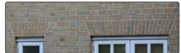
Detail of brick arches
