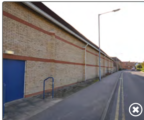
Vast expanse of brick creates a poor environment - Huntingdon
