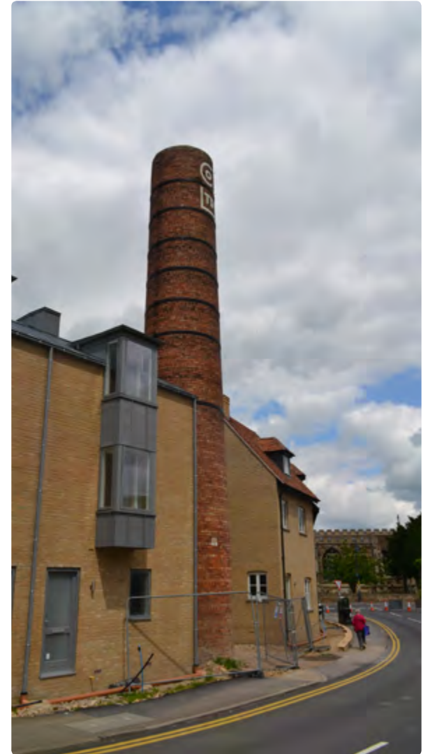
Retention of chimney in new development
