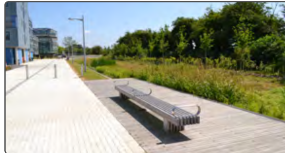
Drainage channel following pedestrian route
