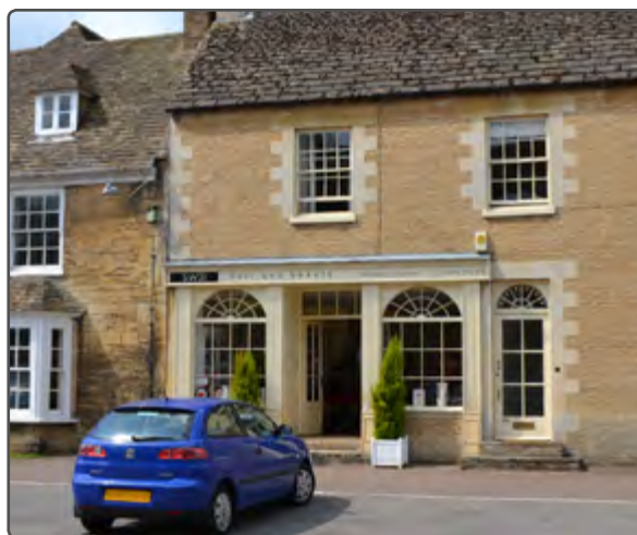
Beautifully proportioned shop front - Wansford
