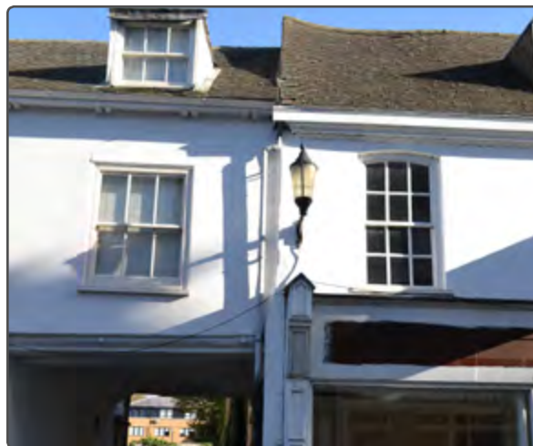
Street light in a good location
