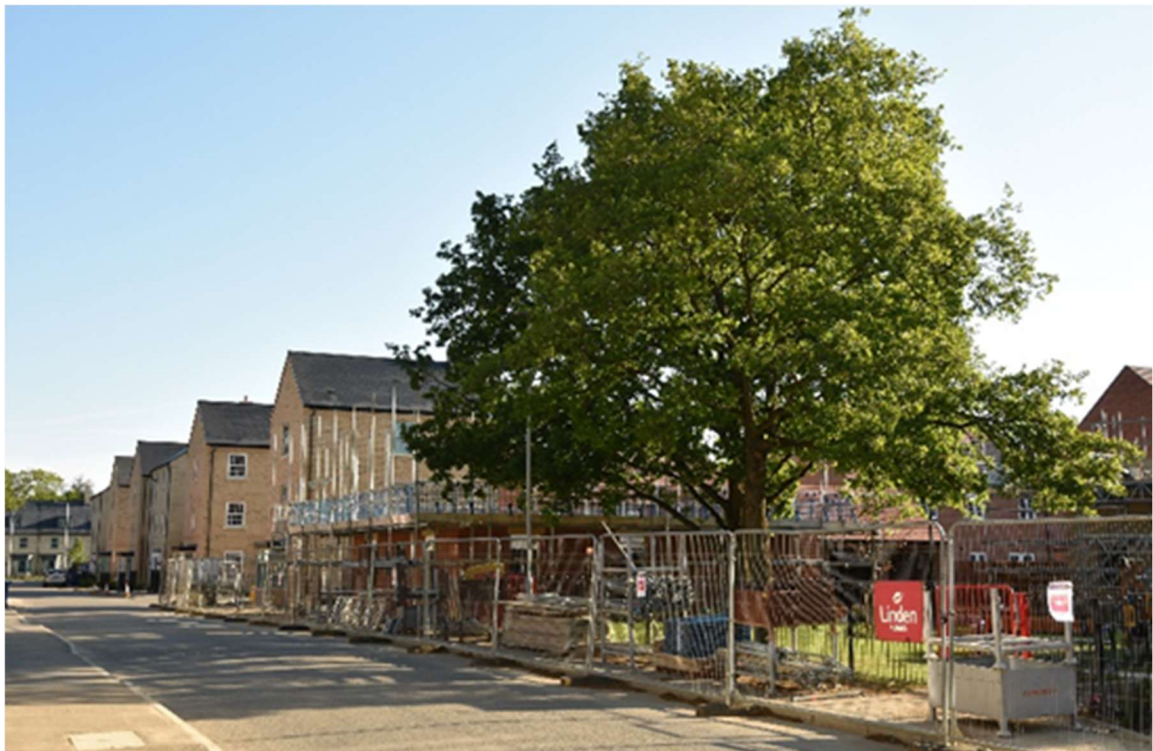
Forster Road, Brampton (HDC)
