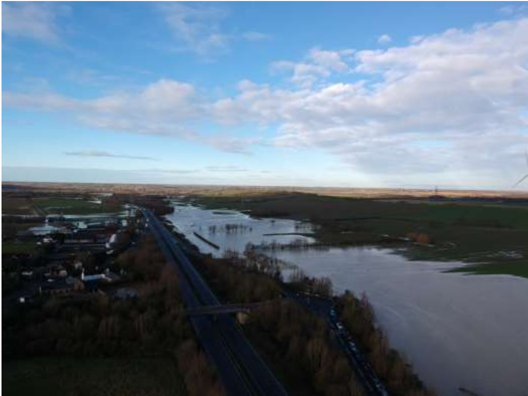
Figure 55: Flooding to the North of the A14, looking West
