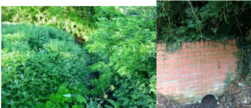
Figure 63: Drains becoming blocked again in Ellington in June 2017
