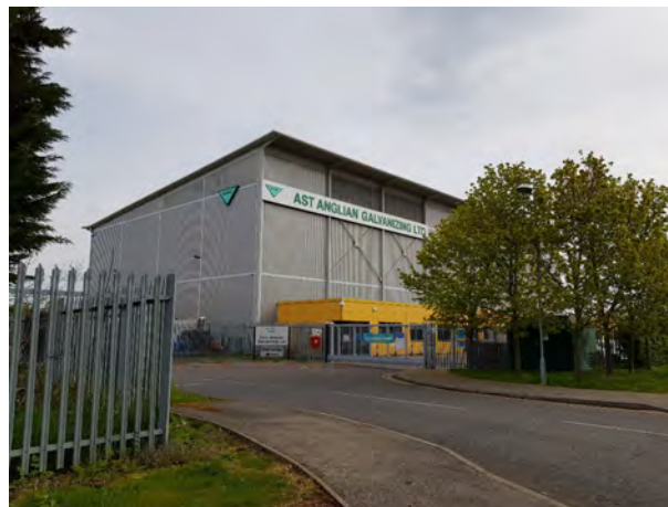
Large factory/industrial unit to the north of Nordic House
