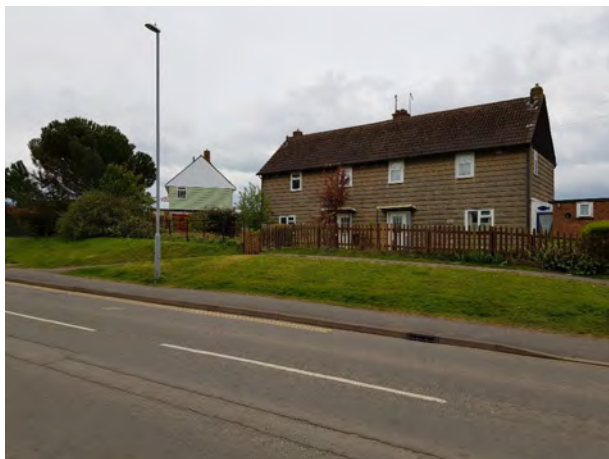
Semi-detached weatherboarded homes along Fen Lane located on raised ground
