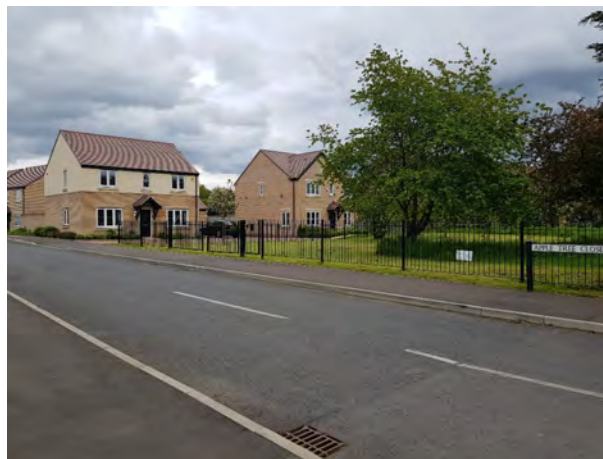
Apple Tree Close properties facing onto amenity space, this also provides a substantial set back from Cambridge Road
