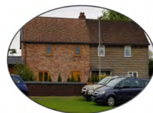
Property where concrete panels have been replaced
