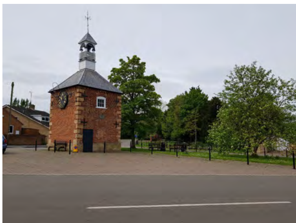
The listed Clock Tower and Lock-up forms a focal point to the village and a memorable approach into the village from Huntingdon Road
