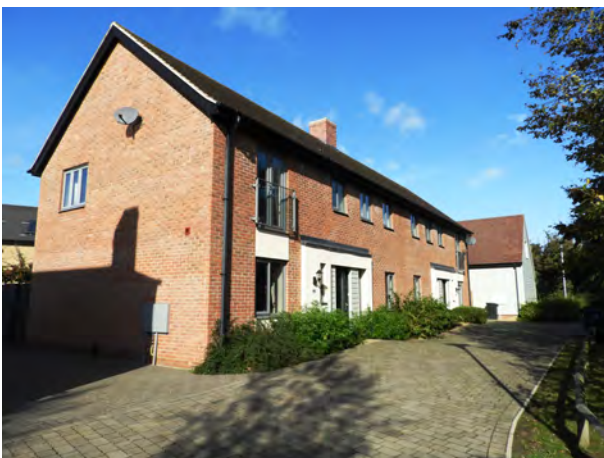
Lodge Drive exemplifies 21st century redevelopment of former industrial land within the centre of the village
