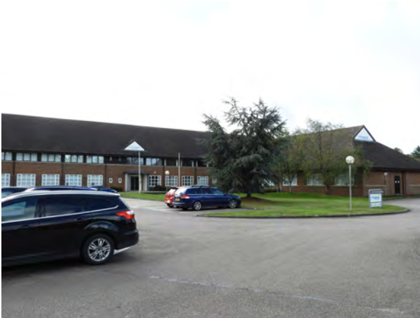
Enterprise House provides significant employment opportunities within a spacious laid out office complex
