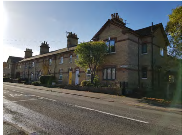
Terraces located along Stukeley Road
