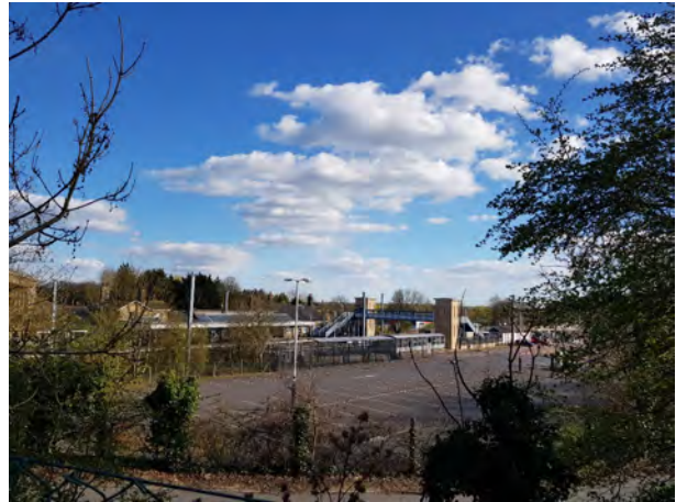
Huntingdon train station
