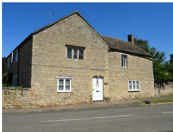
Old Mill House in Elton typifies the use of limestone and Collyweston slates of older buildings in the area
