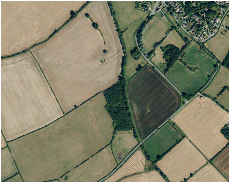
Northern Wolds landscape character area includes a series of ridges and well vegetated valleys with dispersed historic villages
