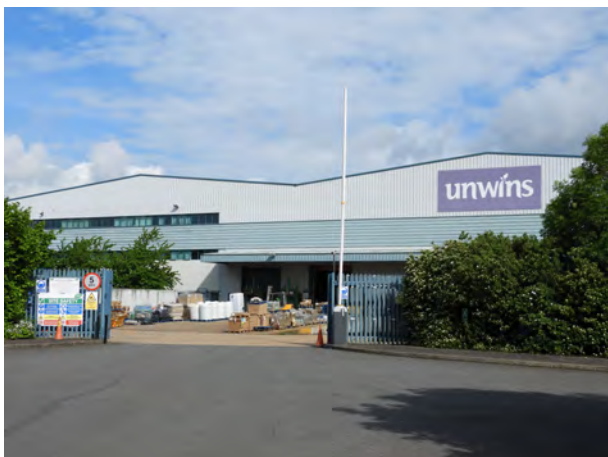
industrial unit at Alconbury Hill
