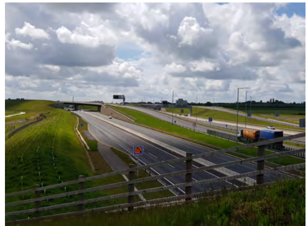
View of the A1 and A14 from overpass looking southwards
