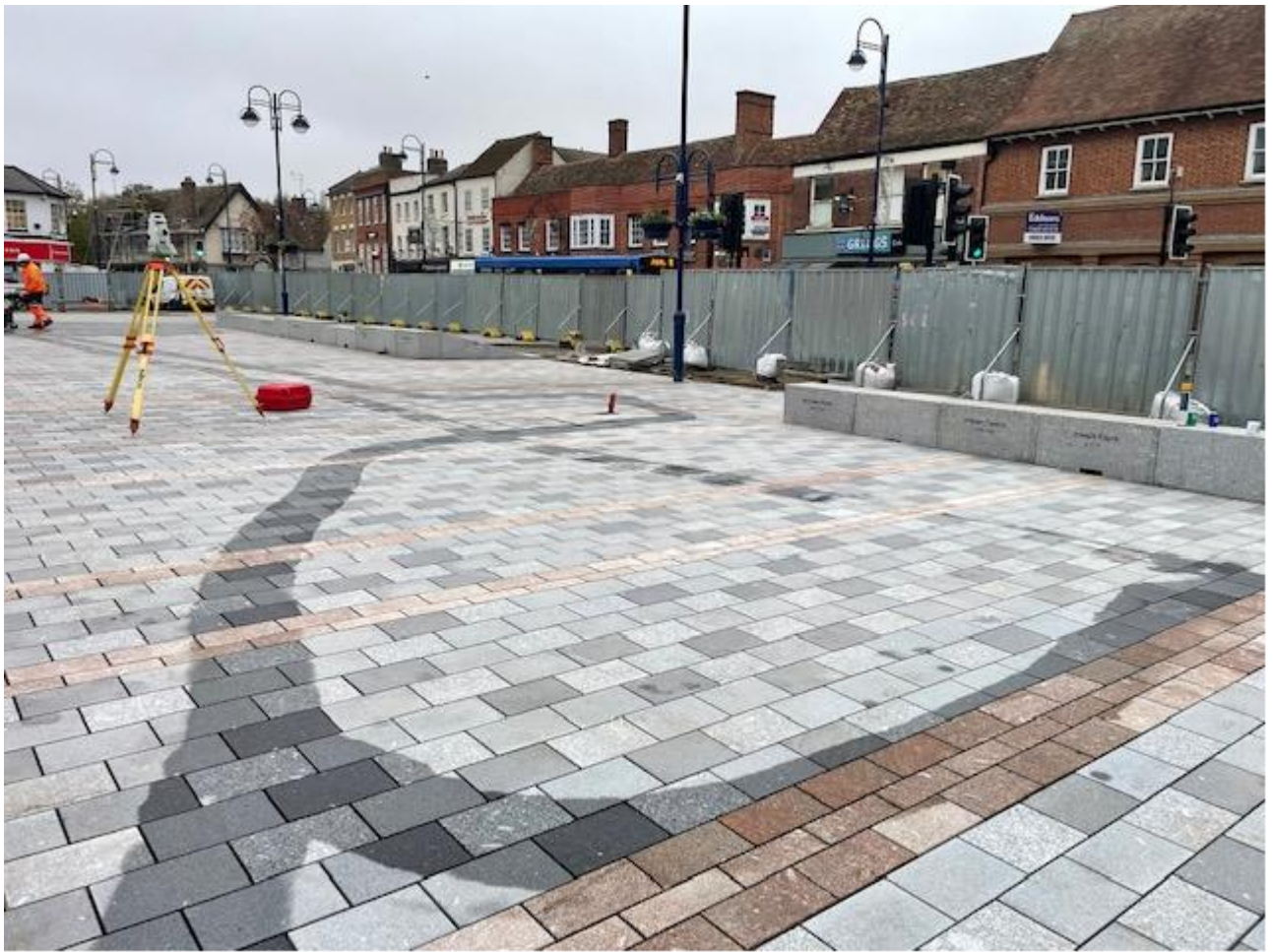
06/11/24 – Market Square blockwork and rain gardens on Market Square north
