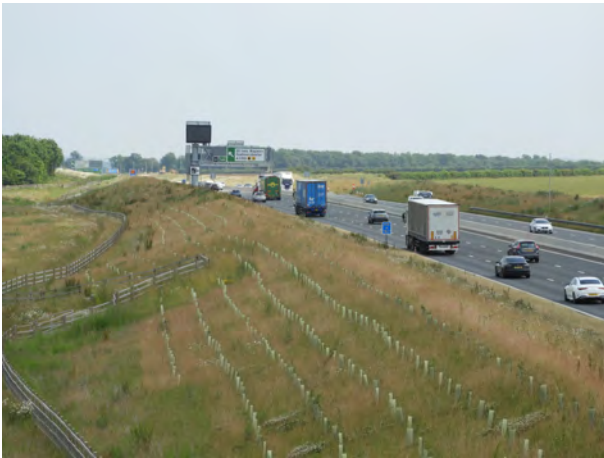
The A14 southern bypass cuts through the area adding extensive planting to soften the impact over time
