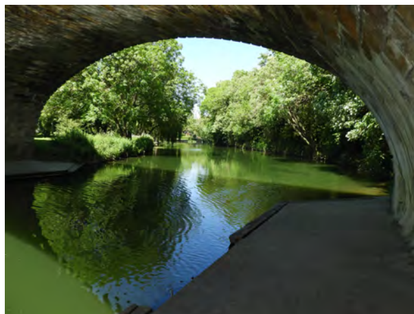
River Nene under the bridge at Wansford
