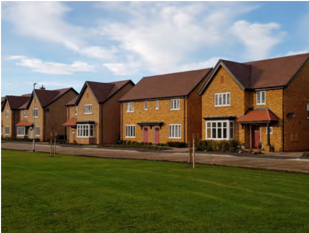
Lucks Lane development in Buckden is the most significant addition to the village providing a mixture of house types and sizes with 21st century design principles while reflecting the local vernacular of buildings
