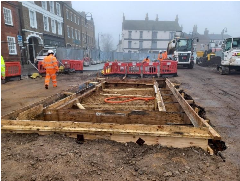
06/02/2025 – Shuttering constructed for rain garden 5 concrete foundation pour
