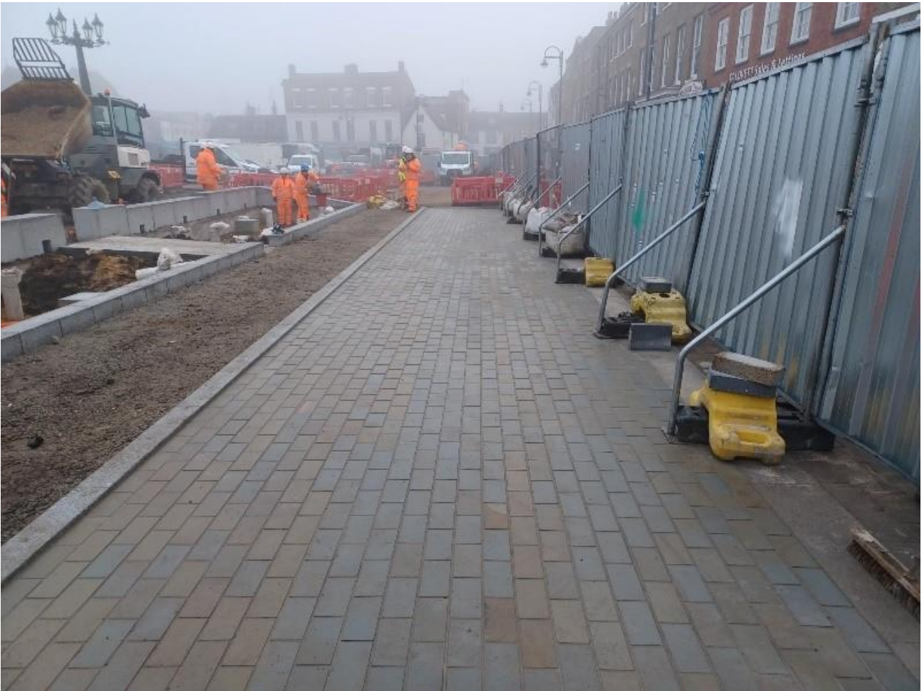
06/02/2025 – First disabled parking layby laid, rain garden 4 blocks installed
