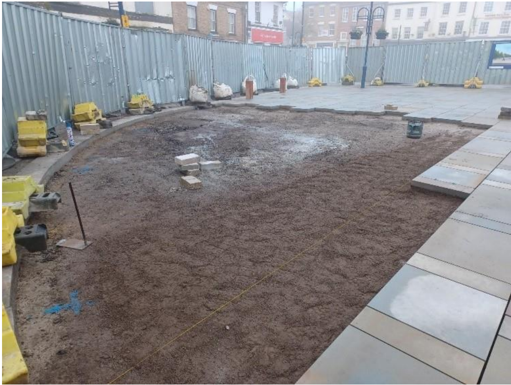
06/02/2025 – York stone slab laying progressing on western side of Market Square
