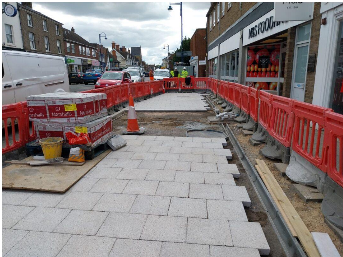
19/06/24 – Paving works outside M&S nears completion
