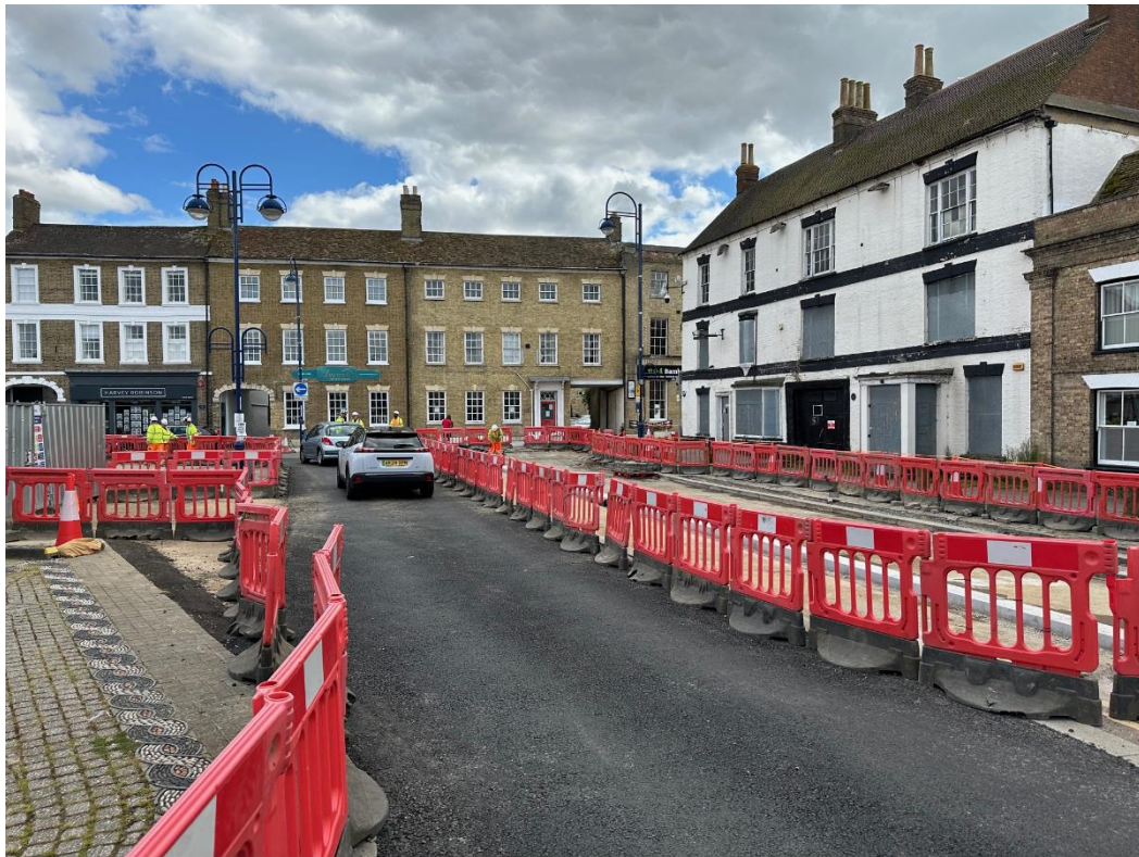
19/06/24 – Temporary road constructed to allow access during resurfacing works
