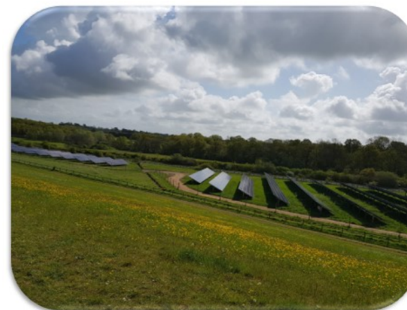
Solar panels near Grafham Water
